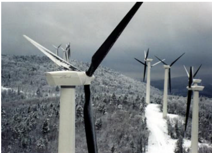
Figure 5. Searsburg turbines use black blades to prevent ice accumulation. Note the layer of ice along the blade leading edge. (National Renewable Energy Laboratory)
