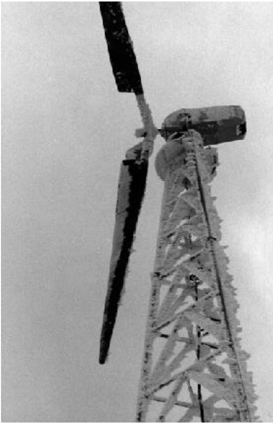
Figure 1. Severe rime ice accretion on a US Windpower 56-100 turbine installed on Mt. Equinox Vt. Note the magnitude and extent of the ice coverage. (University of Illinois at Urbana-Champaign, Dept. of Aeronautical and Astronautical Eng.)
