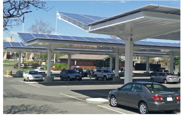
Fig. 1. Solar canopy parking lot with EV chargers.
