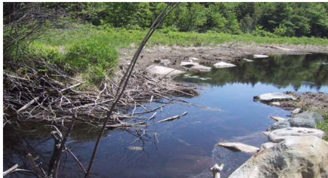
Figure 5.27 Breached dam in Alder Brook (June, 2005)
