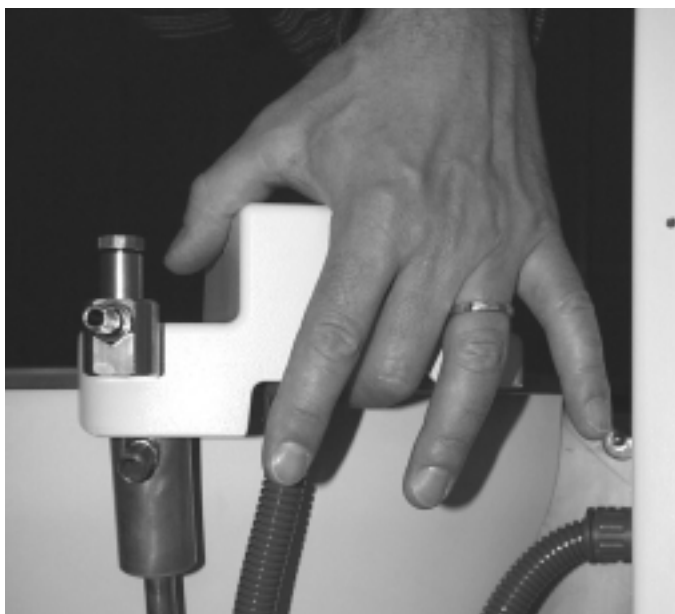
Fig. 22: Reset of the over-temperature protection
