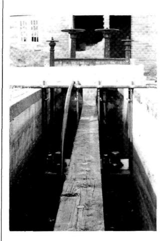
Figure 2. Submersible Raw Sewage Pumps
