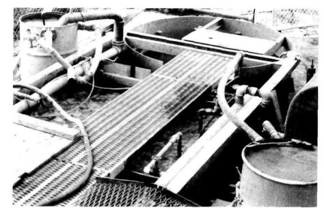
Figure 4. Two-Stage Activated Sludge Pilot Plant (second stage)
