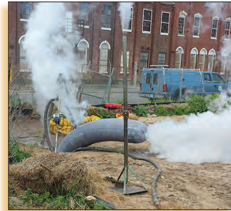
Contractor crews working on Walnut Street
