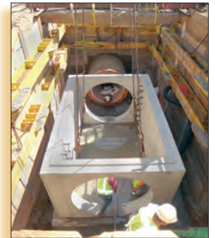
Installation of flow control structure to a sewer main within Arch Street
