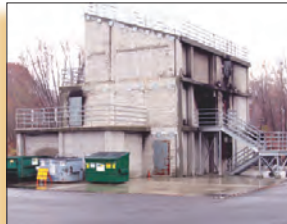
Burn Building at Western Massachusetts Fire Training Facility (photo courtesy of mass.gov)
