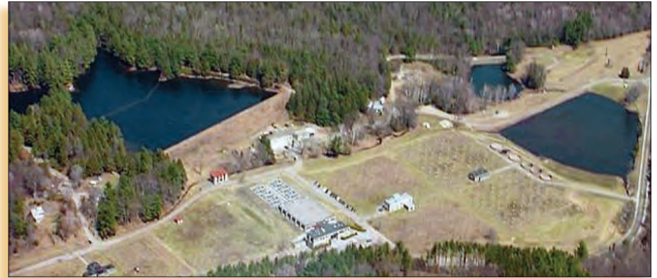
Aerial View of the West Parish Filters Water Treatment Plant
