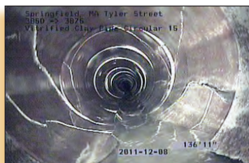
Interior of a sewer main in Springfield obtained as part of the ongoing Collection System Assessment Program
