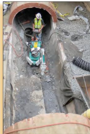
Preparation of an 84-inch sewer for slip lining a new 72-inch pipe within Washburn Street
