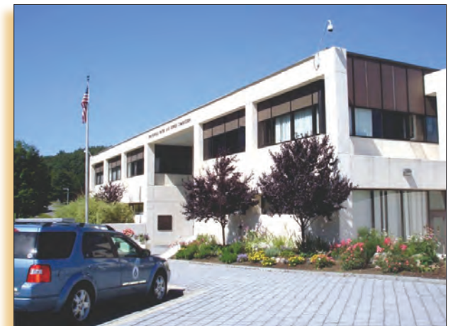
West Parish Filters Water Treatment Plant
