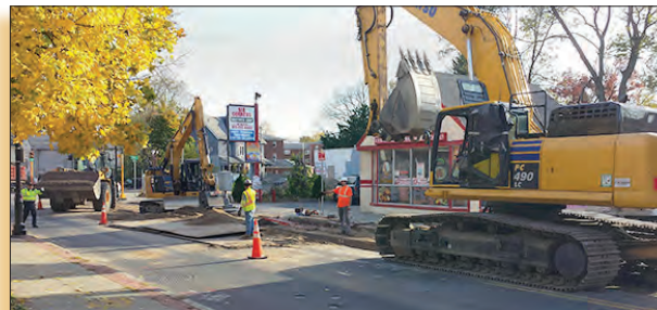
Contractor crews working on Walnut Street
