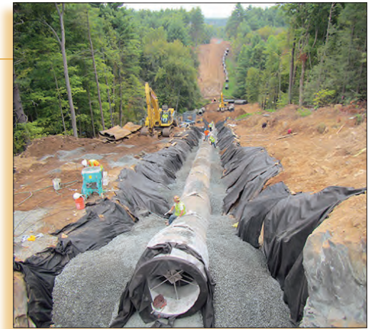
First section of 54" pipe installed
