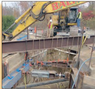
Excavation for a new drain within Birnie Avenue while supporting an active sewer main
