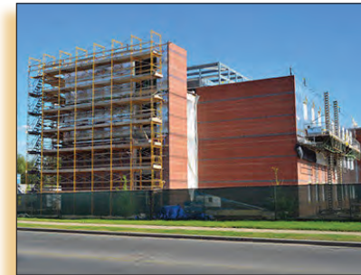
Central High School Construction (photo courtesy of Masslive)
