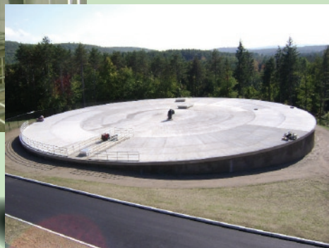
Finished Water Clearwell
