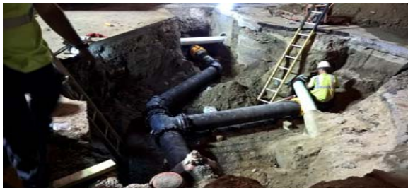
New Water Main, Conz St.
