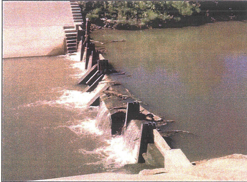
Raising the height of the reservoir on the Delaware River located near the water treatment plant, Kickapoo Tribe in Kansas.
