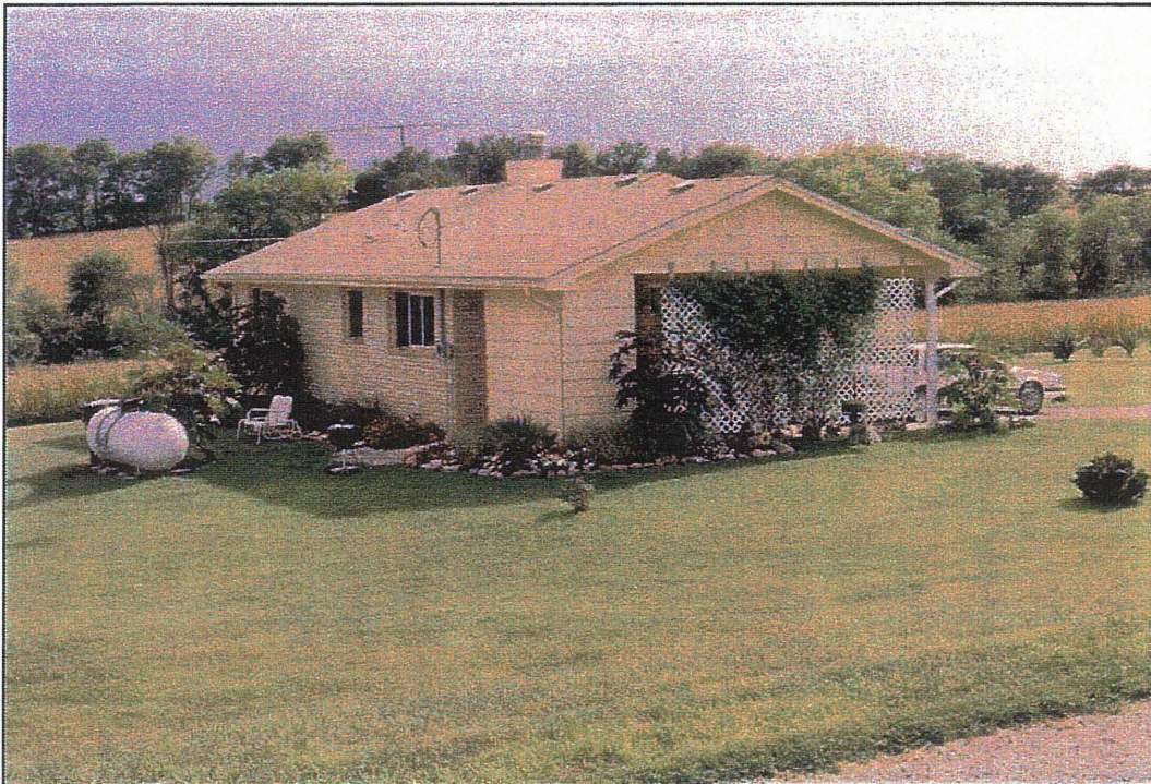
Home in the Red Earth housing area of the Sac and Fox Nation of Missouri.
