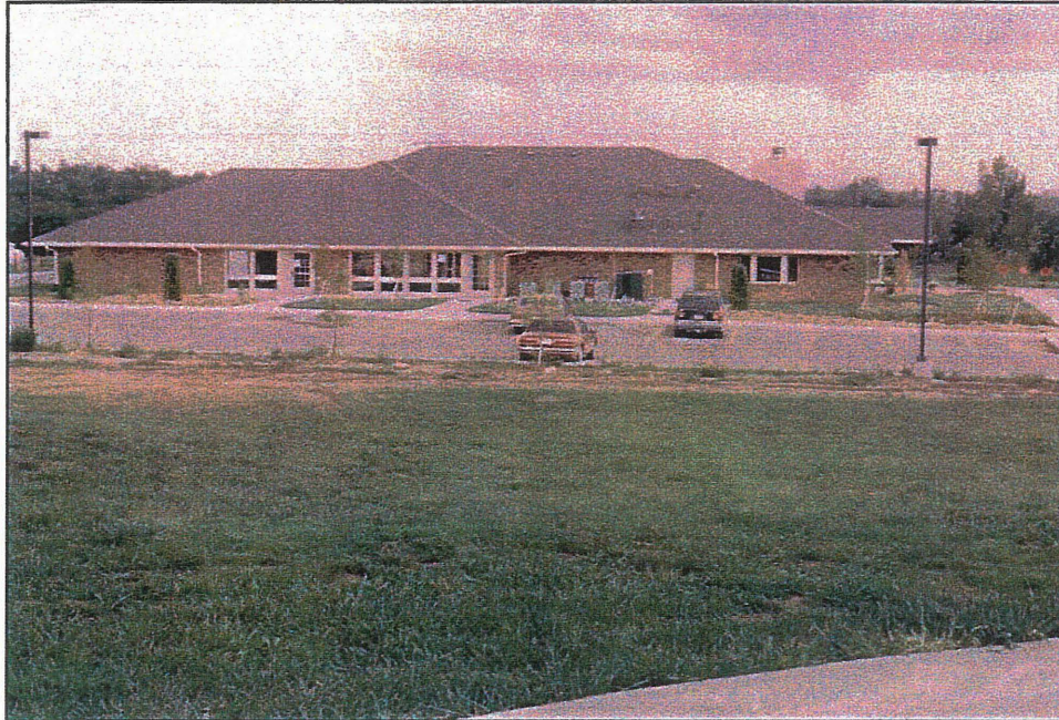
Newly constructed Prairie Band Potawatomi Nation Senior Center.
