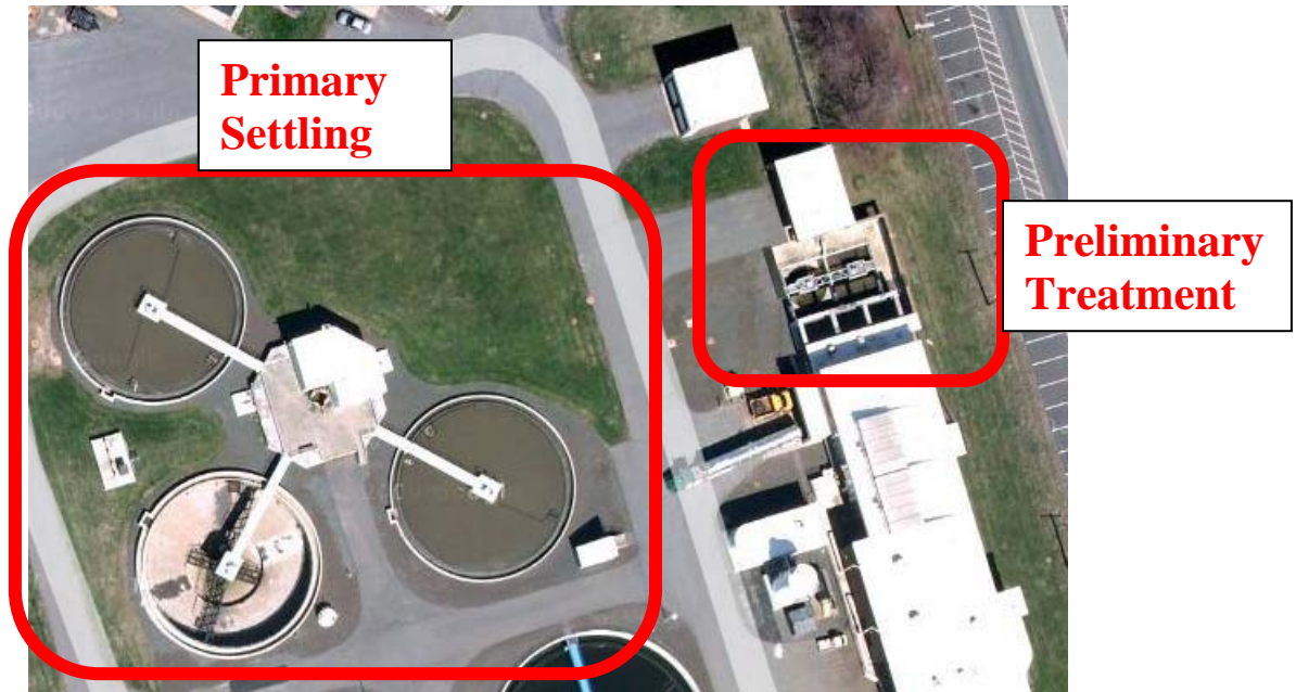
Figure 4. North End of plant showing 3 Primary Clarifiers and Preliminary Treatment Building
