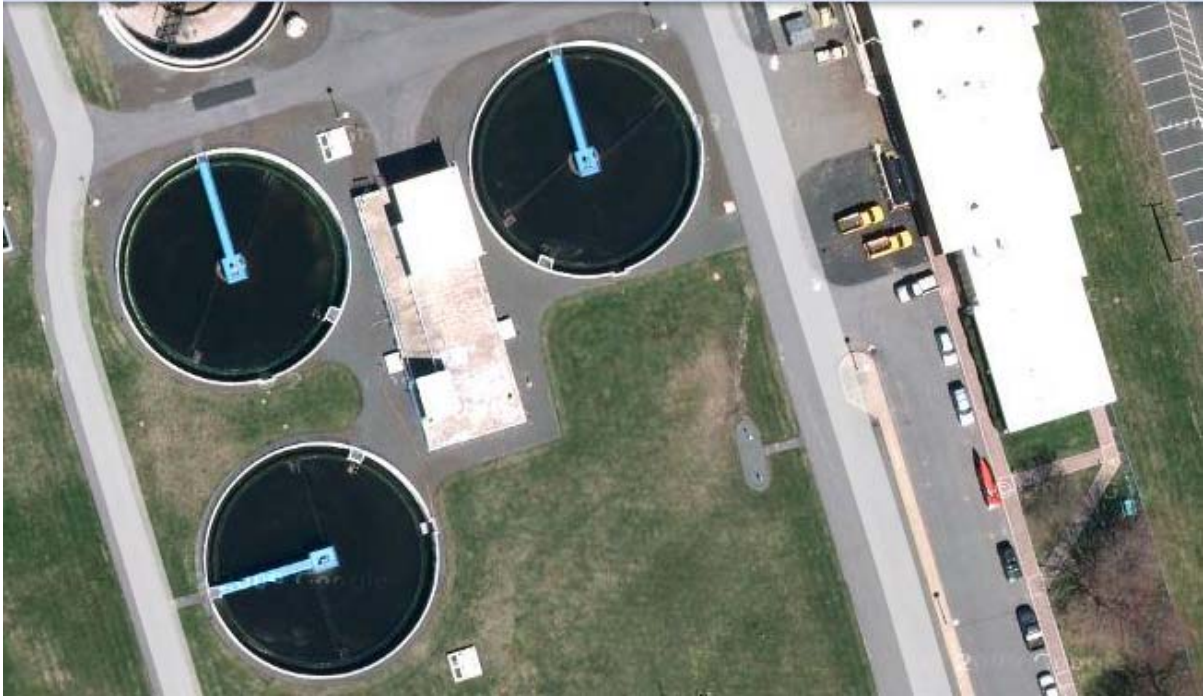
Figure 8. Aerial View of Secondary Clarifiers
