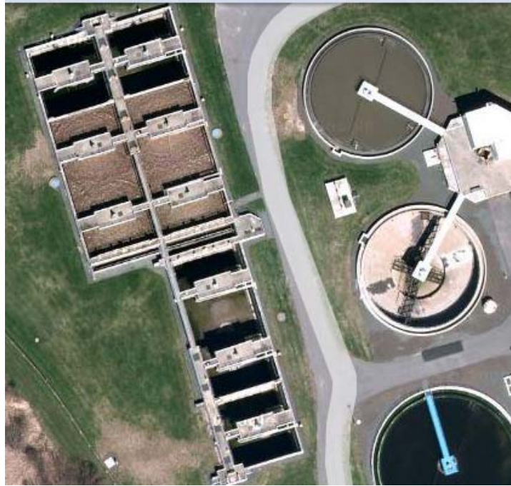
Figure 6. Aerial View of Activated Sludge Tanks (on left).
