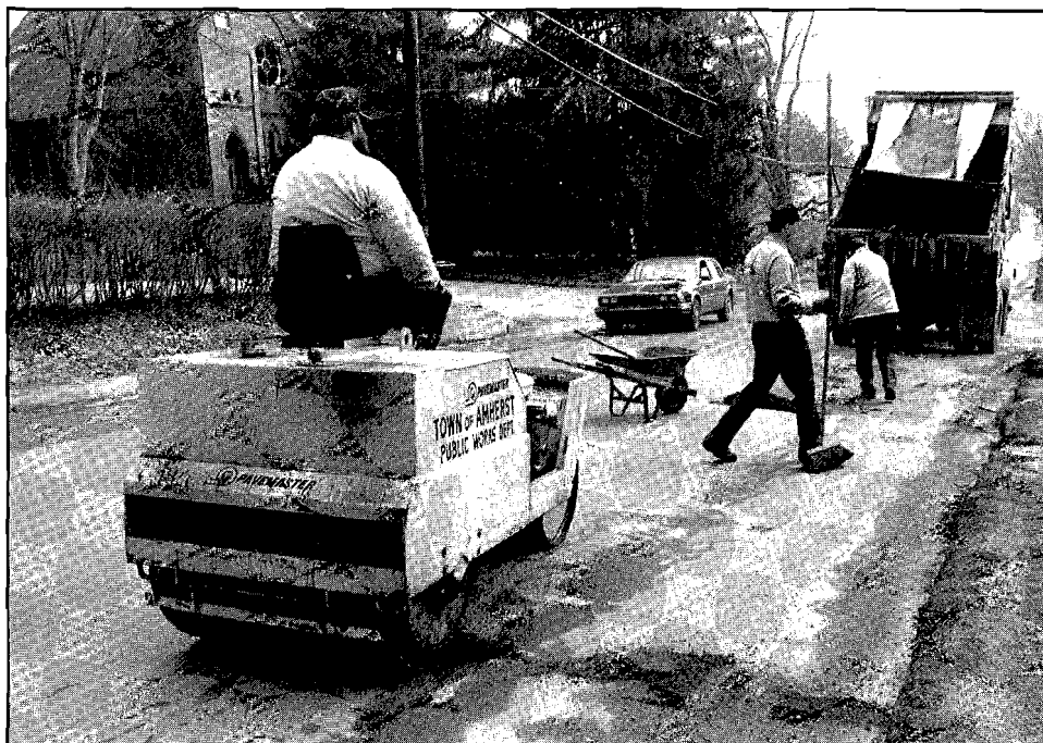
Pothole Patching in Amherst
