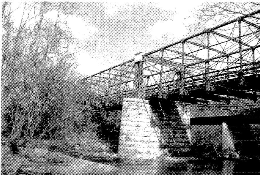
Fig. 1 Bollman truss bridge now located at Savage, Maryland. All photographs by Liakos Ariston.
