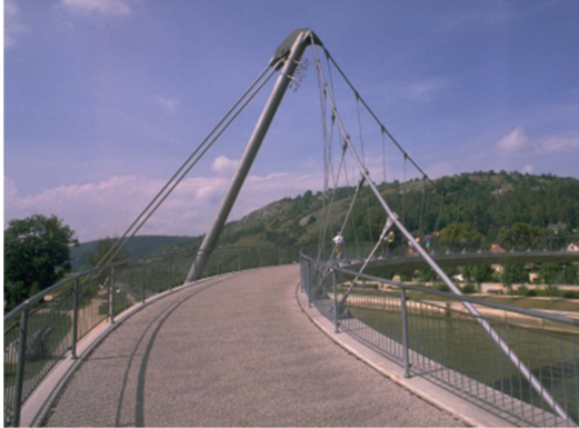
(a) Kelheim bridge (Credit: SBP)
