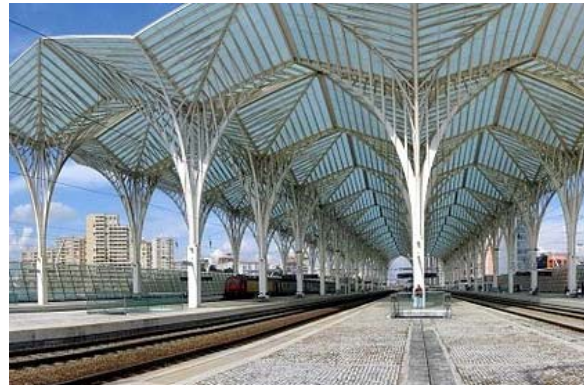
(b) Oriente Station (Credit: Joao Pimentel Ferreira)
