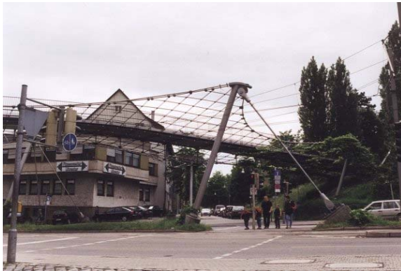
(b) Lowentor bridge (Credit: Nicolas Janberg)
