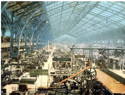
(a) Galerie des Machines (Credit: Library of Congress)
