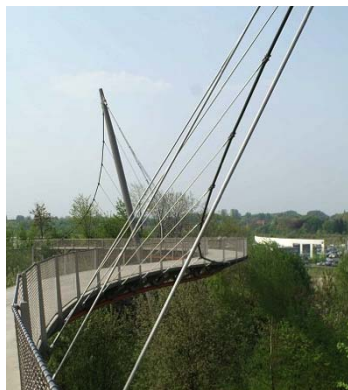
(c) Gahlensche Strasse bridge (Credit: Nicolas Janberg)
