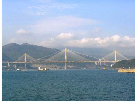
Figure 5: Ting Kau bridge (Credit: Baycrest)
