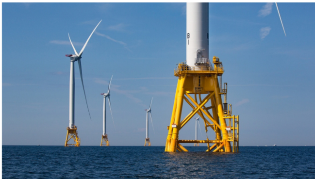
Fig. 3. Block Island Wind Farm support structures (image courtesy Z. Finucane, Keystone Engineering).
