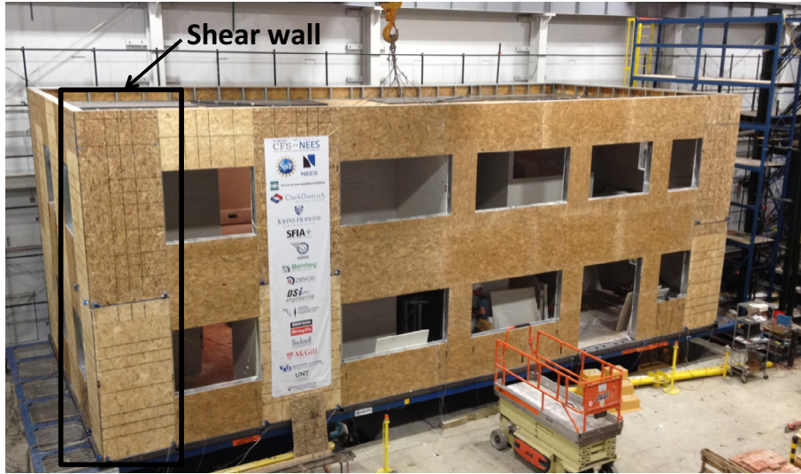
Fig. 1. CFS-NEES building and shear wall in it.
