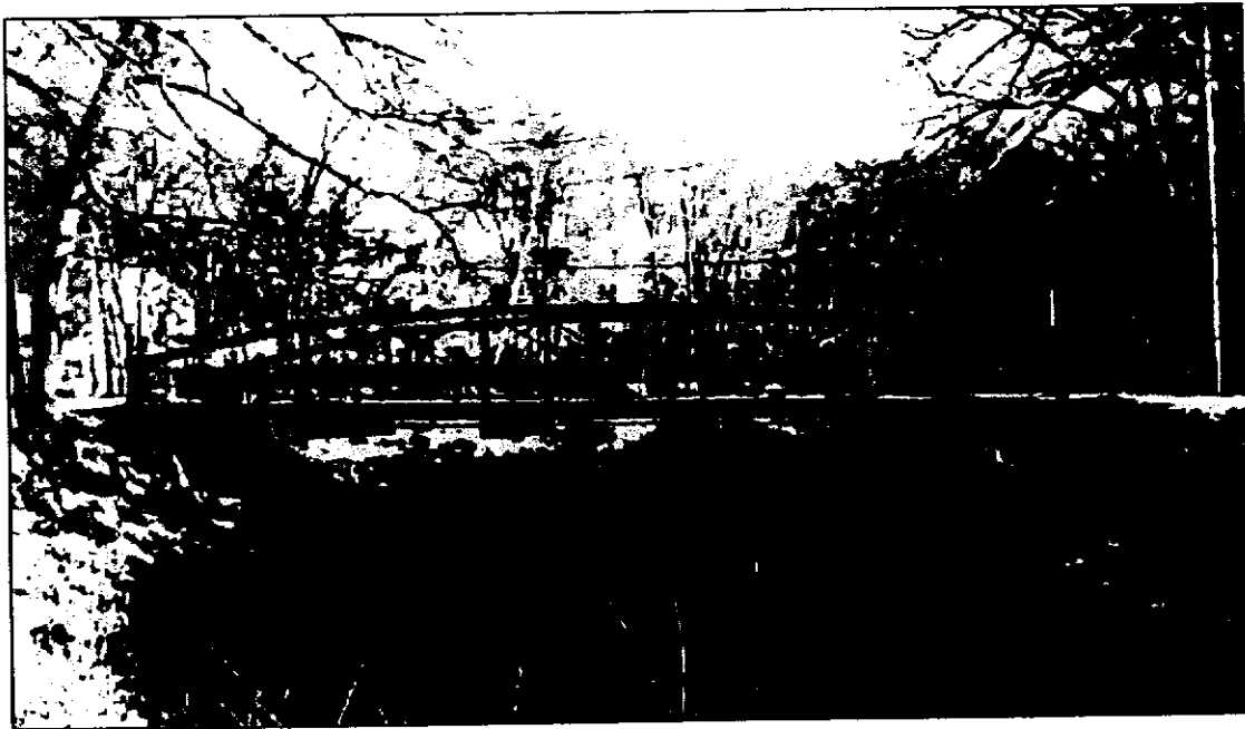
FIGURE 14. The Gilbert Road Bridge in West Warren.
